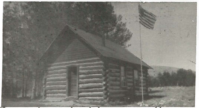
Log cabin school house at Morrison Creek.
