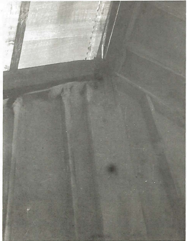
Foam Insulation sprayed on walls
