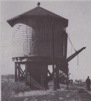
Rio Grande railroad water tank in the Gunnison railroad yard about 1950. This was Gunnison's second water tank. Built in 1924, at a cost of $3,524.55, it was dismantled in 1955. (Photographer unknown, from the author's collection)
