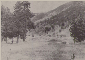
View along old Colorado and Southern grade, continuing (behind camera) to Graymount, and line of Argentine Central coming in from the right. Scars of side-hill cuts at two levels show on Pendleton Mountain in background. The two railroads joined at this site.
