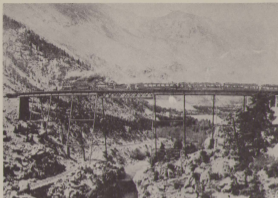
Real bridge, phantom train. Good faking but some errors show. The Georgetown Loop was always featured as a part of the Argentine Central package. Edward B. Wilcox.
