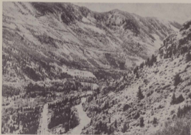
Argentine Central switchbacks on Pendleton Mountain. Georgetown Loop tracks in foreground. Edward B. Wilcox.
