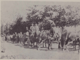
Teams hauled supplies to Waldorf before the Argentine Central was built. Edward B. Wilcox.
