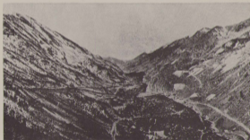
Argentine Central grade rises on Pendleton Mountain from Silver Plume. Georgetown Loop in right foreground. Site of accident on grade to left.
