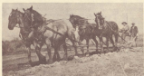
Walt Aldridge and Jim Keller working on the county road one-half mile north of Cedarvale, 1913.
