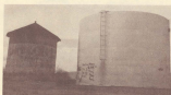
The original water tank built in 1916 for the Orchard City water system on the left and the tank built in 1950. They were constructed on the hill, southwest of the Orchard City town hall.
