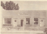
Cedaridge Town Hall built in 1931. Mrs. Blanche Phillips, long time town clerk is in the doorway.
