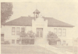
Eckert High School built in 1902. The high school closed in 1945 and the building was used for Eckert Elementary grades. 1945 grades one, two and Kindergarten meet at the school.
